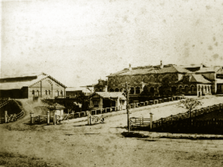
c1880, Roma Street Railway Station, viewed from Roma Street. (JOL 712)
